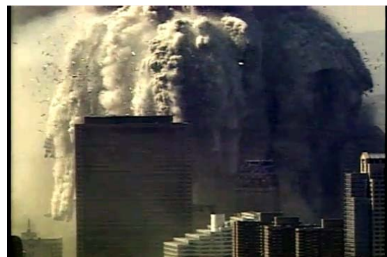
Note the large, free-flying steel framing sections, trailing smoke clouds, which landed hundreds of feet outside of the building's perimeter.
