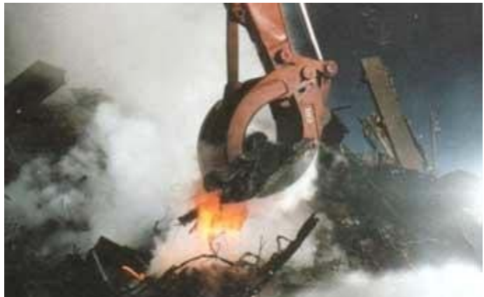
An excavating machine at Ground Zero lifts debris dripping with molten metal
